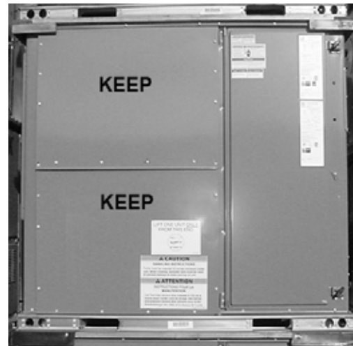
Figure 20: Save Side Panels For Economizer Hood Tops
