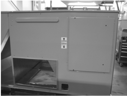
Figure 17: Side Panels With Hole Plugs
