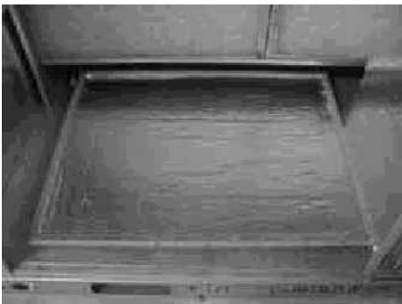
Figure 18: Return Downflow Plenum With Panel
